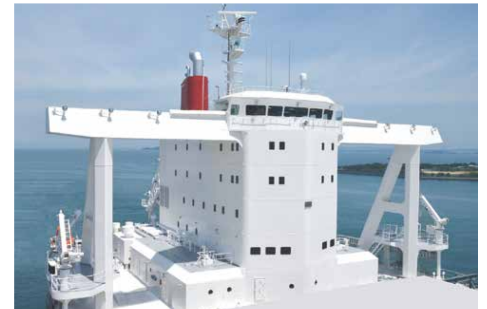
CITADEL on a ship, provided by Imabari Shipbuilding Co. Ltd
